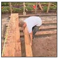
**Sleeper deck:** Nigel a H4 sleeper pine treated deck. The area was levelled using compacted roadbase. The bearers were set out at 1200m then sleepers laid across, staggering the joints and nailing into place.
