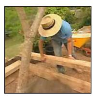
**Planter boxes:** Jamie used sleepers to create planter boxes for the frangipani, making sure of a sound level base to lay sleepers on edge. Our box height was 470mm and this was two sleepers on edge and a capping sleeper laid flat for seating, with the ends cut at 45 degrees to give a mitred finish. *Blitz tipz:* Raised beds improve drainage and are perfect for herb and vegetable plots
